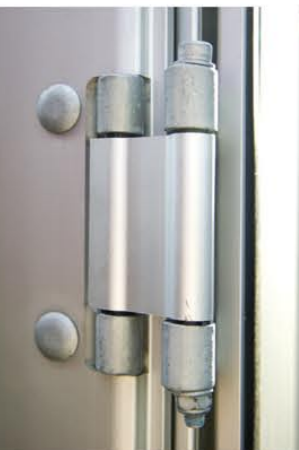
Bearing hinges with plastic slide bushes
